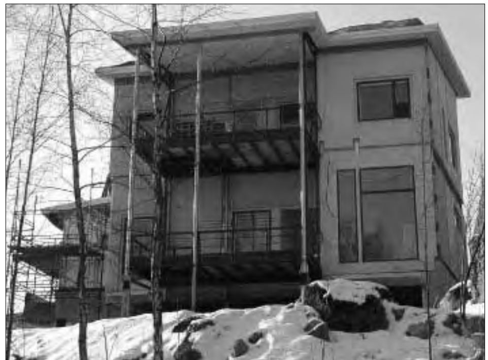
Figure 4. Demonstration industrialized housing construction in Finland.
