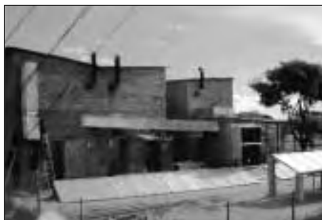
Solar tobacco drying installation at Tobacco Research Station, Zimbabwe.
