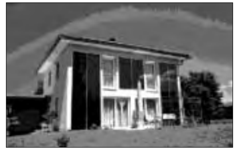
Solar combisystem with 22.7 m 2 façade-integrated collector in Austria
