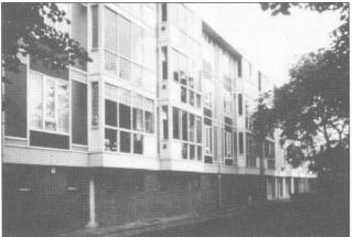
contributed 64 percent of that reduction. A variety of technologies were used both to save energy and to improve these apartments, including air collectors integrated into the south facade for preheating ventilation air, glazed balconies on the south facade, glazed galleries on the north facade, better windows, and additional insulation.
