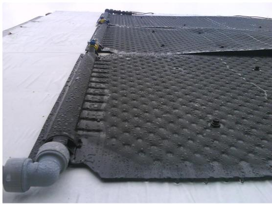
Fig. 3: Close up of the absorber showing the connecting pipe and header along the left side of the collector. The mounting screws to the roof can also be seen. It is assumed while modeling that no large amount of air flow can go behind the collector, so that a one sided operation/condensation can be expected. In a real situation a "two sided" mounting arrangement allowing air behind the collector may increase the performance during low temperature operation. (Photo from SP)
