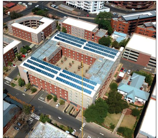
▲ Figure 1. District heating system on the Wits Junction residence building combines solar thermal, co-generation and gas technologies
