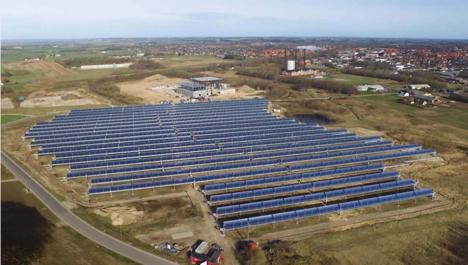
Parabolic trough collector field in Brønderslev, Denmark with an installed capacity of 16.6 MW th supplies not only heat to the district heating network, but also to power production as an add-on to a biomass-fuelled ORC system.
