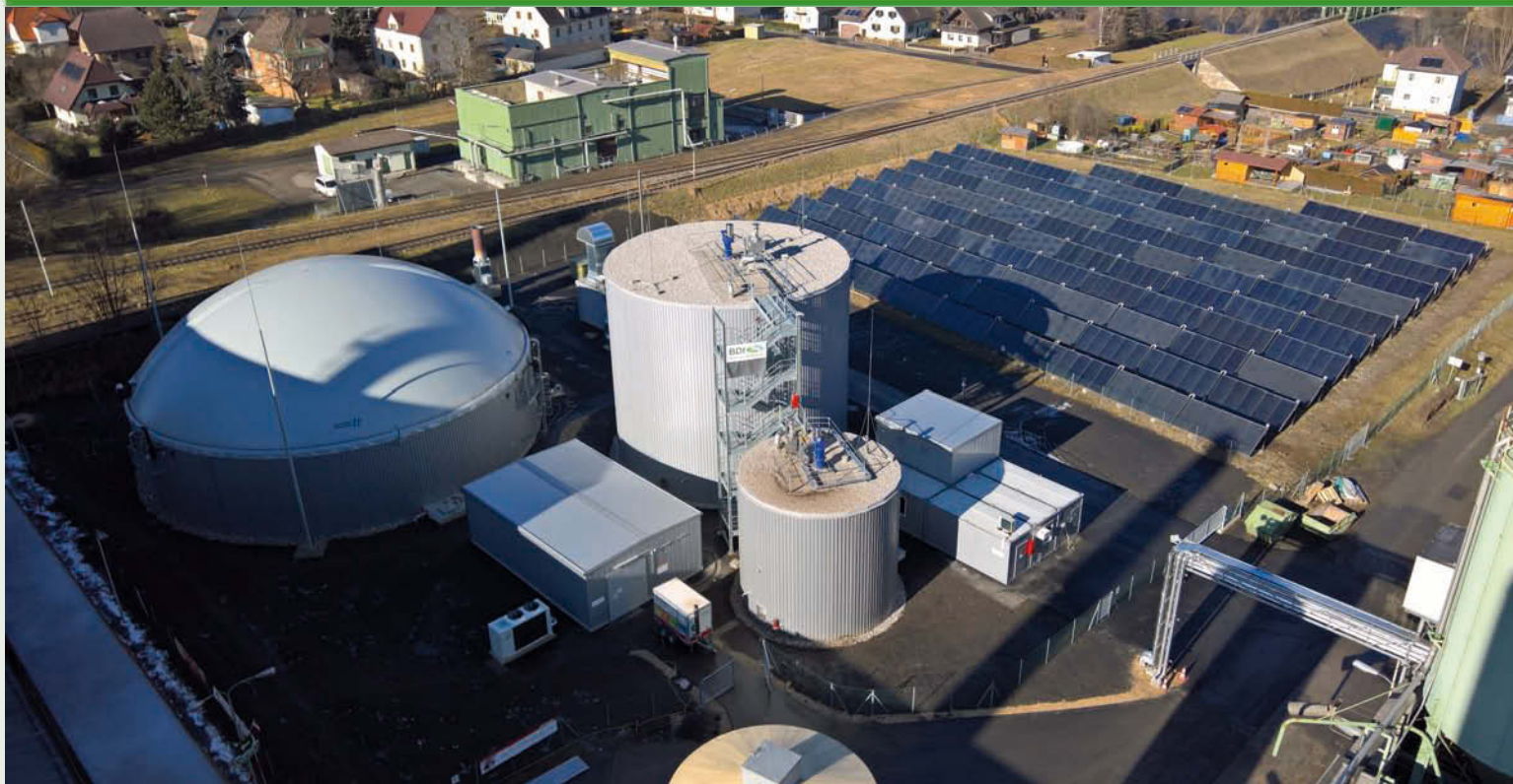
1 MW th solar process heat plant at the Goess Brewery in Austria.
