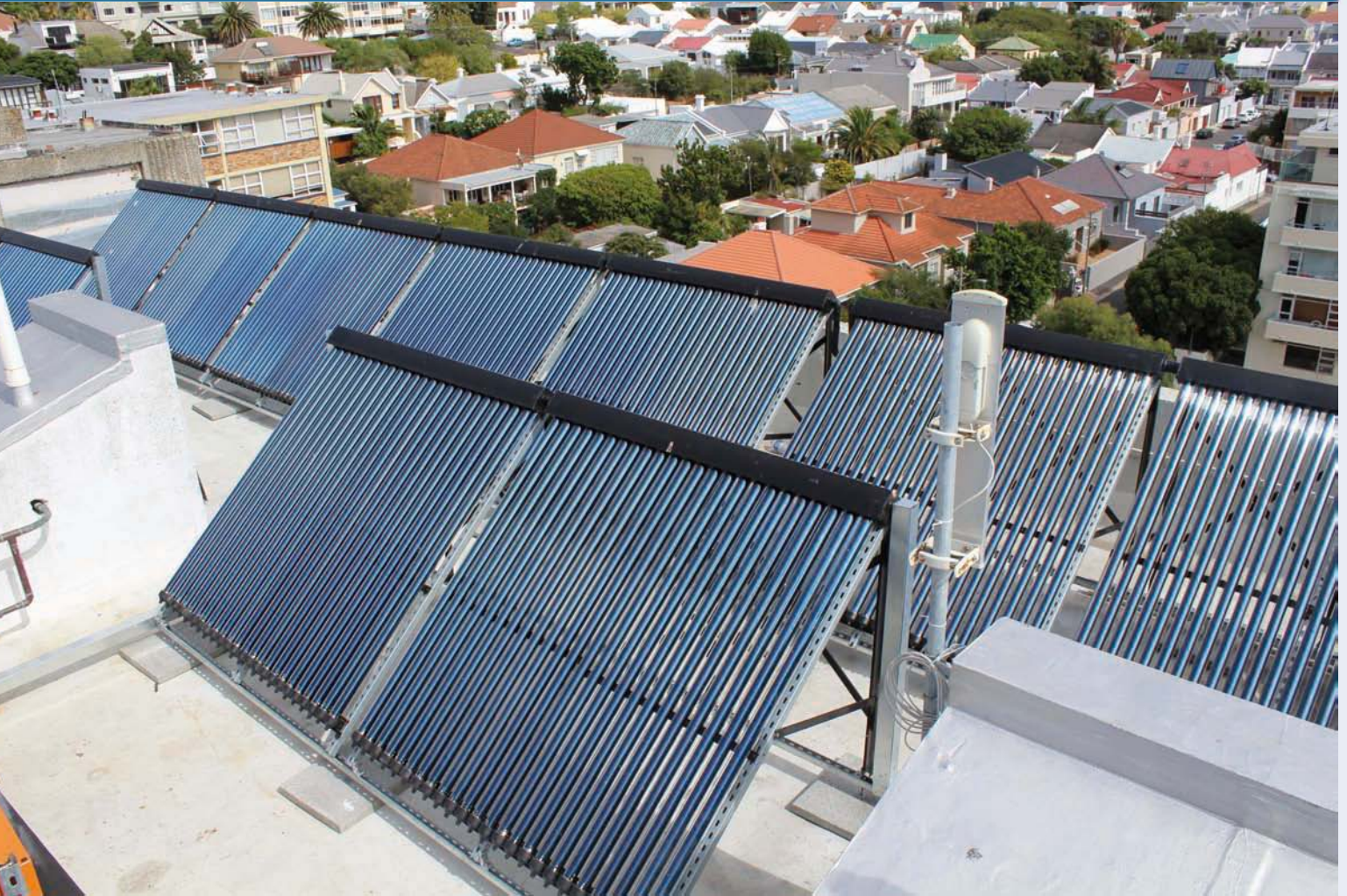
85 m² evacuated tubes at Centurion Building, CapeTown
