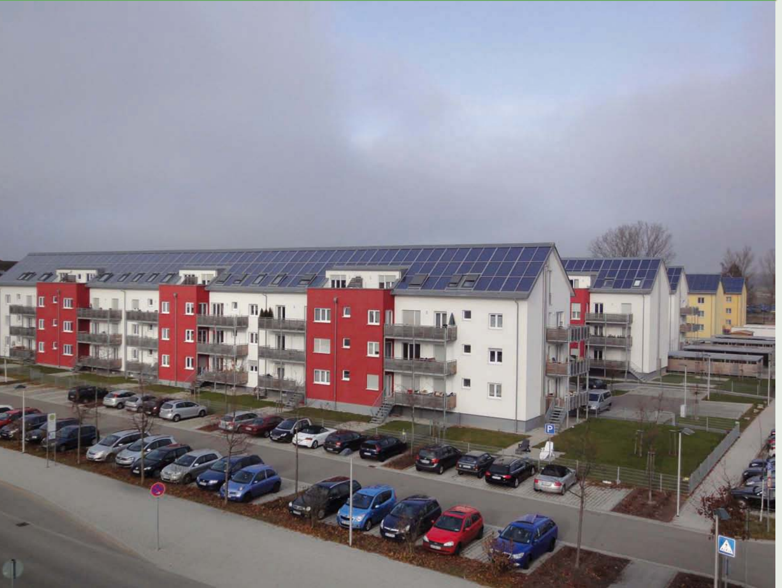
Multi-family buildings in Crailsheim, Germany. Large-scale system with 5.1 MW th installed capacity. Photo: ITW / TZS University of Stuttgart, Germany.
