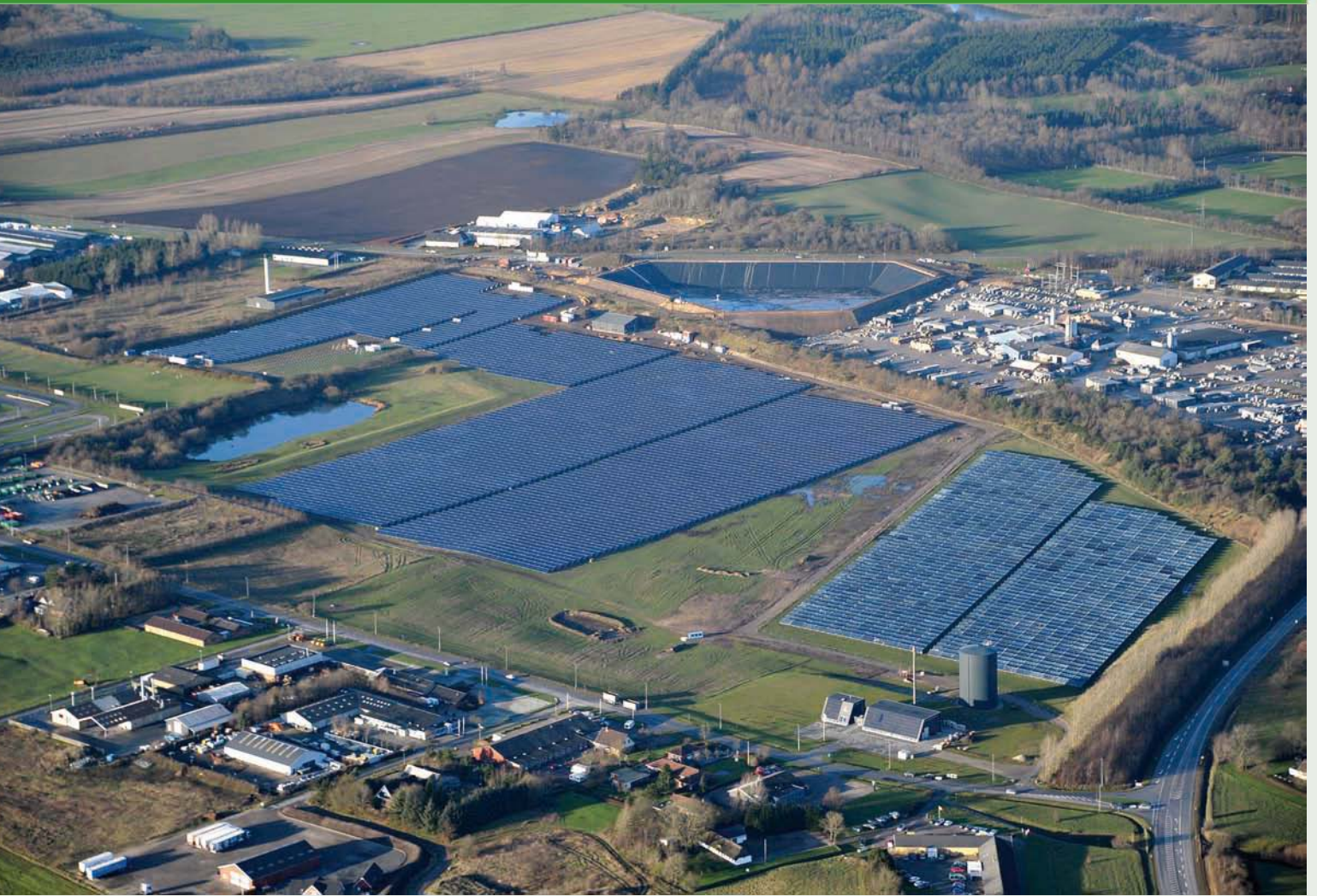
Solar district heating system in Vojens with load-balancing pit storage, Denmark.
