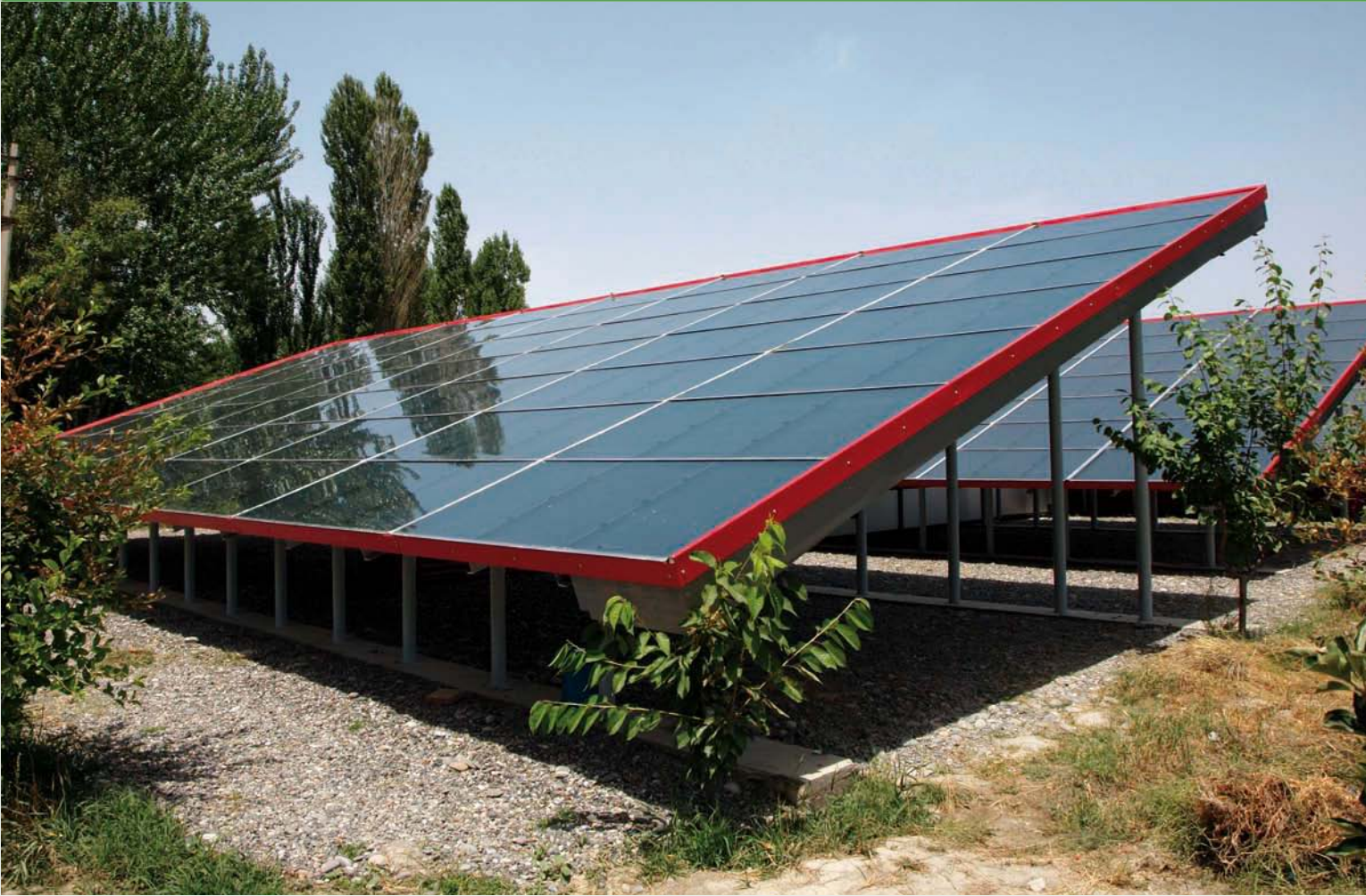
Solar air collector system in Uzbekistan.
