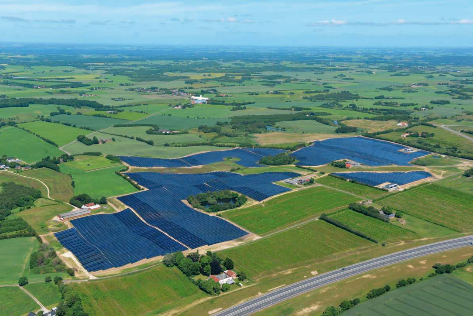
156,694 m 2 solar collector field at Silkeborg, Denmark
