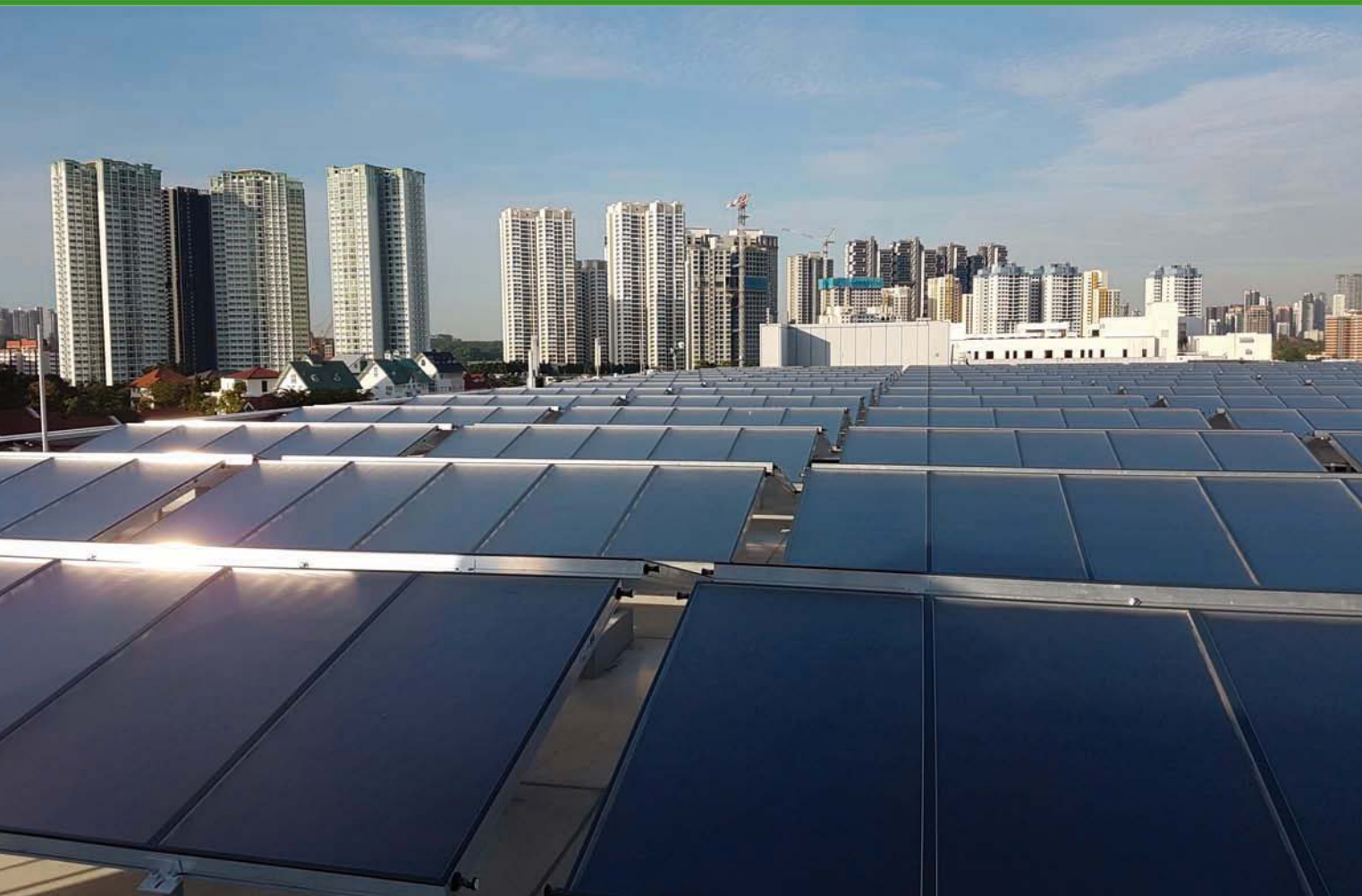
2,472 m 2 solar cooling system at IKEA Singapore delivers 1,587 MWh for an 880 kW absorption chiller.
