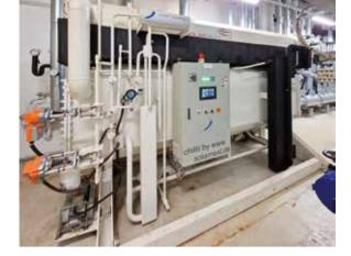
Solar thermally driven 348 kW cooling capacity water/ LiBr absorption chiller for air-conditioning at 16/10 °C chilled water temperature in Mali Photo: Frank Molter, SolarNext
