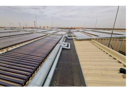
700 m<sup>2</sup> vacuum tube solar collectors supply heat to drive a 348 kW water/LiBr absorption chiller for air-conditioning a new cafeteria and kitchen at Camp Castor in Mali
