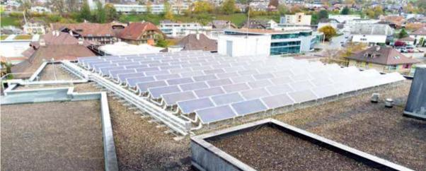
A leading Swiss milk processing company uses 147 kWth (210 m²) of high vacuum flat plate collectors for cheese production Photo: TVP Solar, Switzerland
