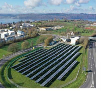
The 4,286 m<sup>2</sup> ground-mounted vacuum tube solar thermal system supports the renewable heat supply for 24,700 residents in Ueberlingen, Germany
