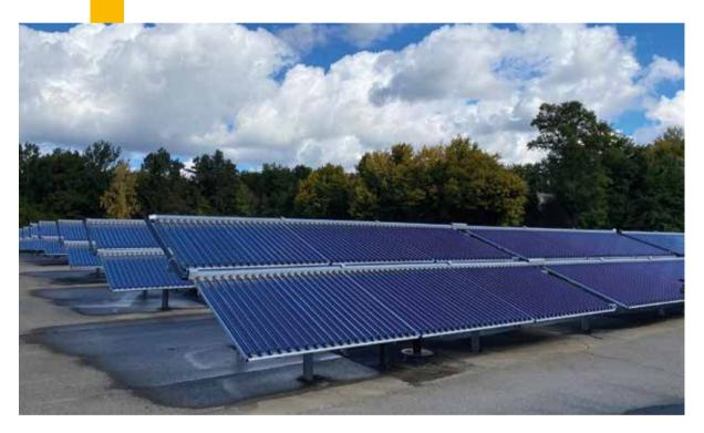
Solar district heating Sigmaringen in Germany with 2,312 m<sup>2</sup> collector area in connection with a 400 m<sup>3</sup> heat storage Photo: Ritter Energie- und Umwelttechnik GmbH & Co. KG
