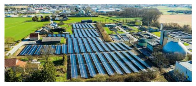
Solar district heating plant in Lemgo, Germany, consists of 9,181  $\rm m^2$  vacuum tube collectors Photo: Stadtwerke Lemgo GmbH / Viessmann
