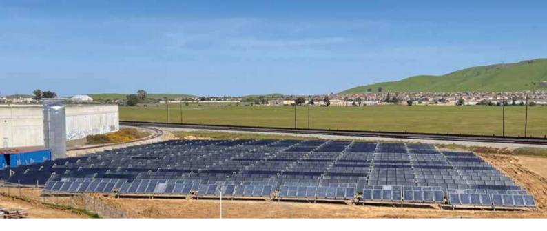
Solar process heat system at the Ball Corporation, headquartered in Fairfield, California, USA. Flat plate collectors with a capacity of 2.8 MW $_{\rm th}$  (3,956 m $^2$ ) provide the heat for washing beverage aluminum cans Photo: SOLID Solar Energy Systems, Austria
