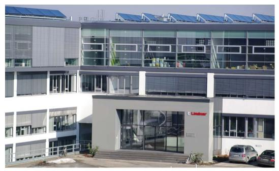
Figure 8: Lindner office building with flat plat collectors on the roof (Source: ZAE Bayern)
