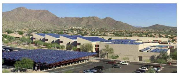
Figure 2: Roof mounted solar collectors at Desert Mountain High School (Source: SOLID)
