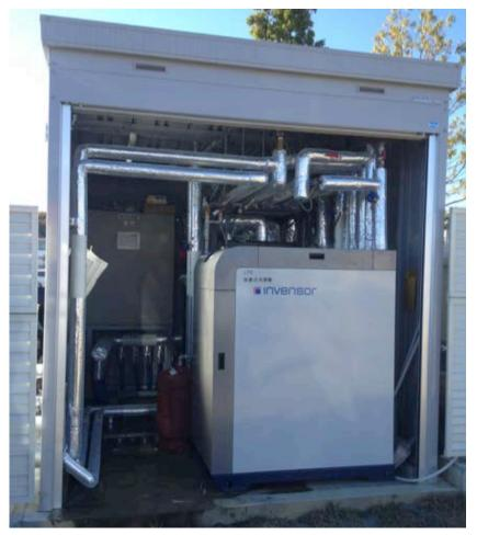
Figure 28: Adsorption chiller of the solar cooling system (Source: InvenSor)
