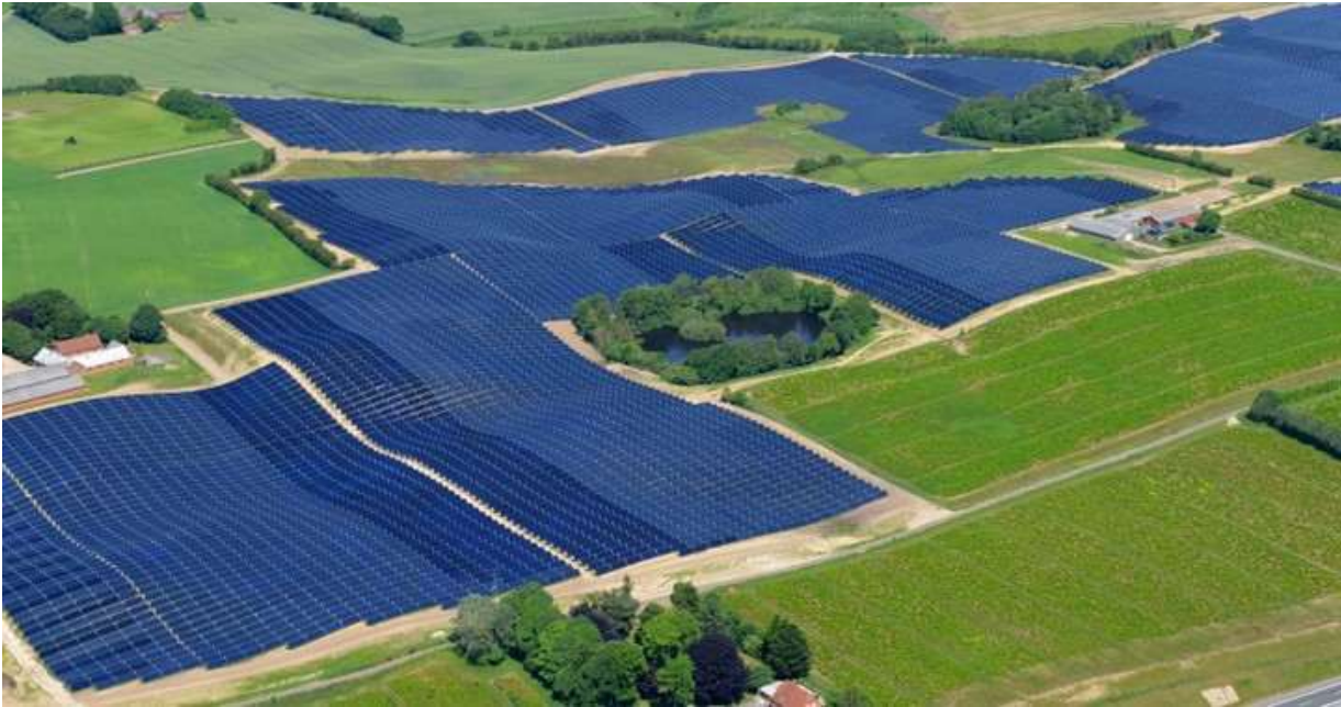
Figure 1 The largest thermal solar district heating plant of the world, in Silkeborg, Denmark
