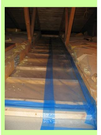
Tightening of the vapour barrier towards the attic
